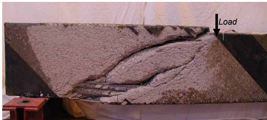
Fig. 7: Typical failure pattern of strengthened beam, 245W, with CFRP removed.
