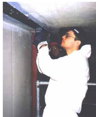
Figure 4-4: Bonding of laminate
