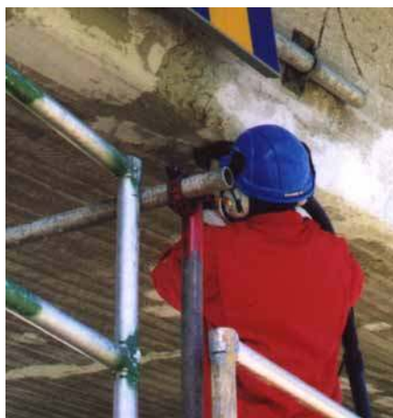
Figure 4-1: Grinding of putty repair of an old damage from vehicle impact
