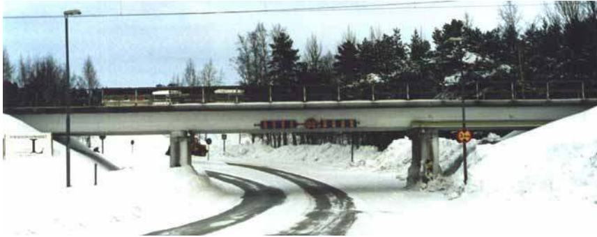
Figure 4-5: The Kalkällan Bridge during winter season, (Täljsten and Carolin, 1999)
