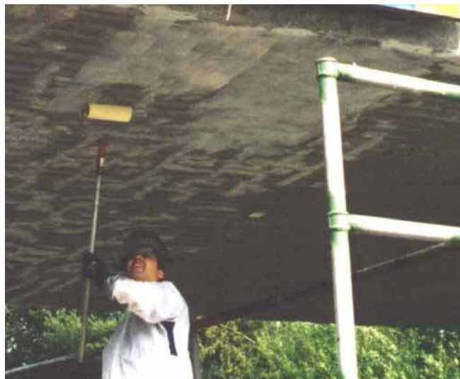
Figure 4-2: Application of primer to the clean and smooth concrete surface.
