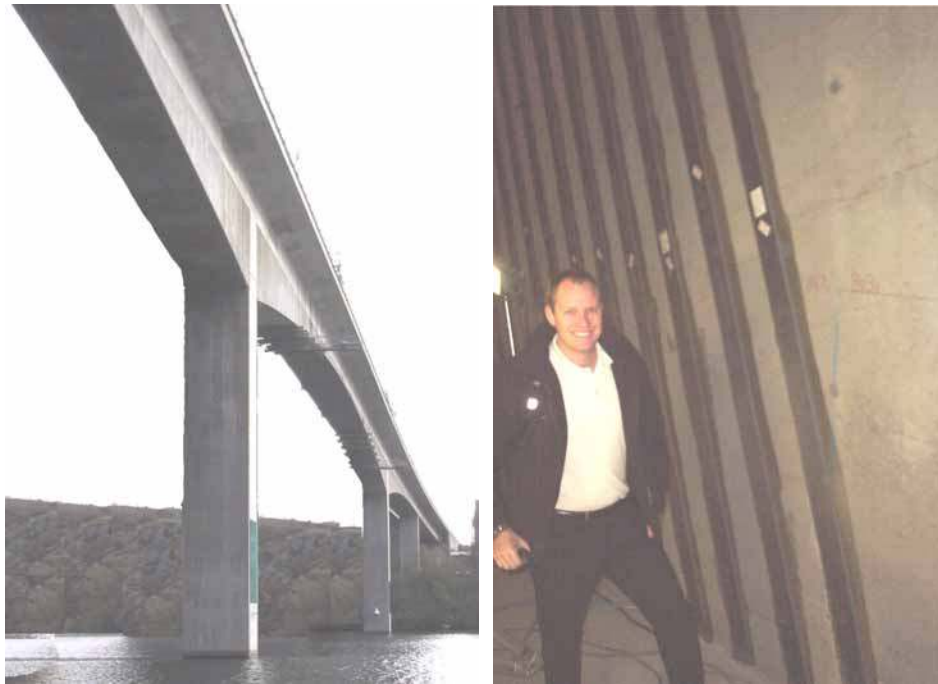
Figure 4-13: Gröndal Bridge. Outside (left), Inside (right).
