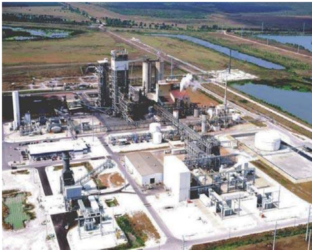
Polk Power Station: IGCC Plant in Tampa, FL (250 MW)
