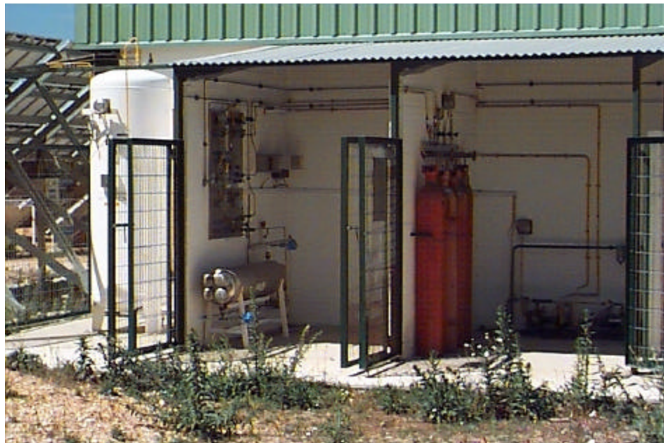
Picture 6.3: Storage System: intermediate buffer (left), horizontal hydride container tank (middle), and 200-bar bottle and compressor (right).
