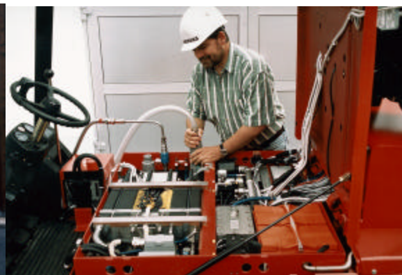
Picture 1.6: PEM fuel cell plant
