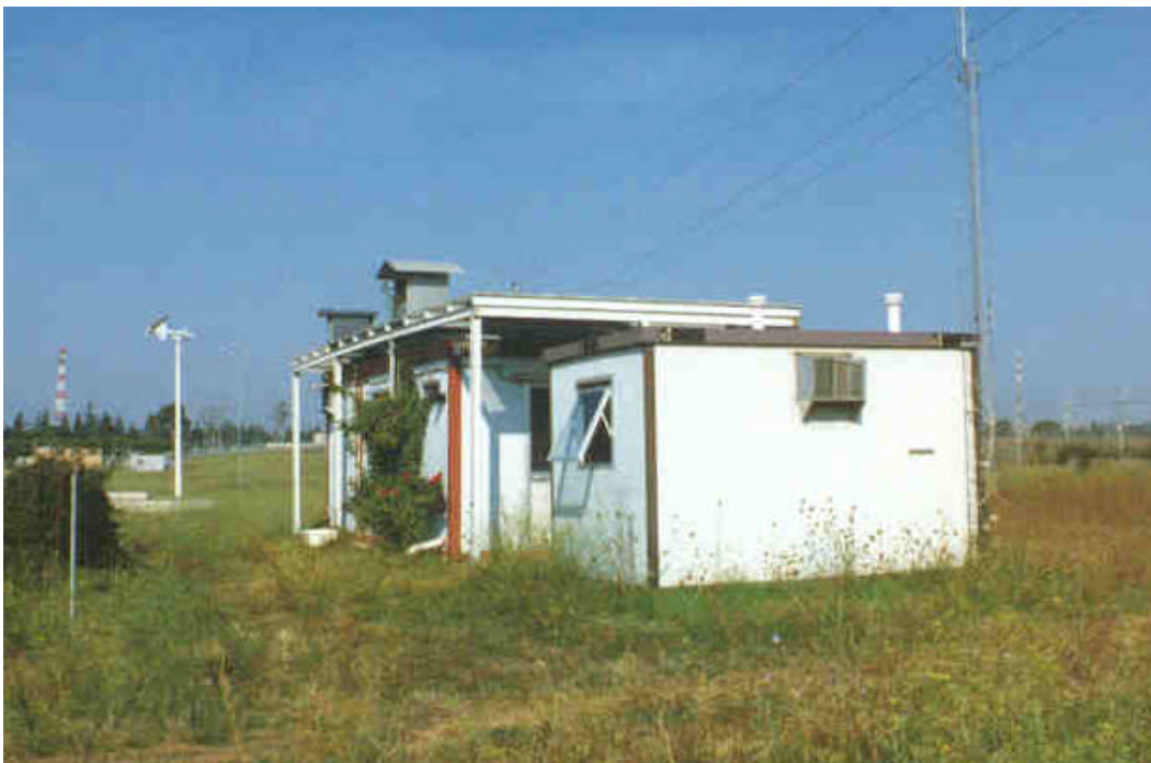
Picture 9.3: Project Site at ENEA Casaccia
