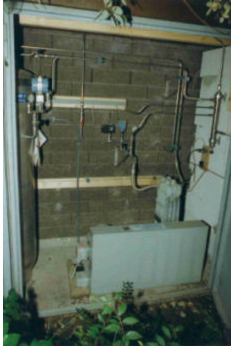
Picture 2.5: Compressor and intermediate storage vessel (partial view on side of picture).
