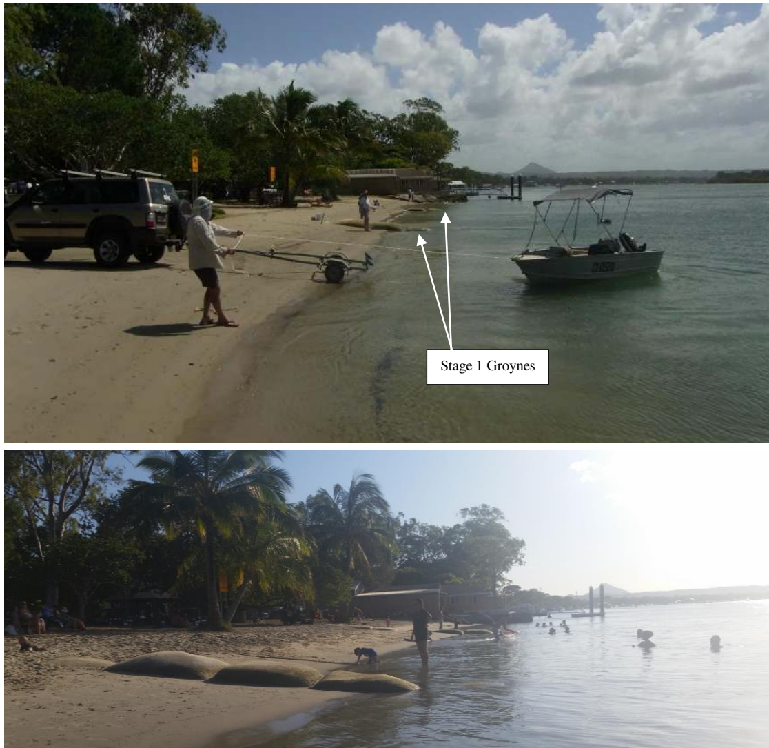
Figure 14. Beach Usage and Low Visual Impact after construction of Stage 1
