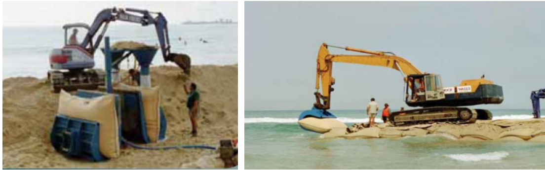
Figure 7. Traditional Method of Filling Sand-Filled Geotextile Containers
