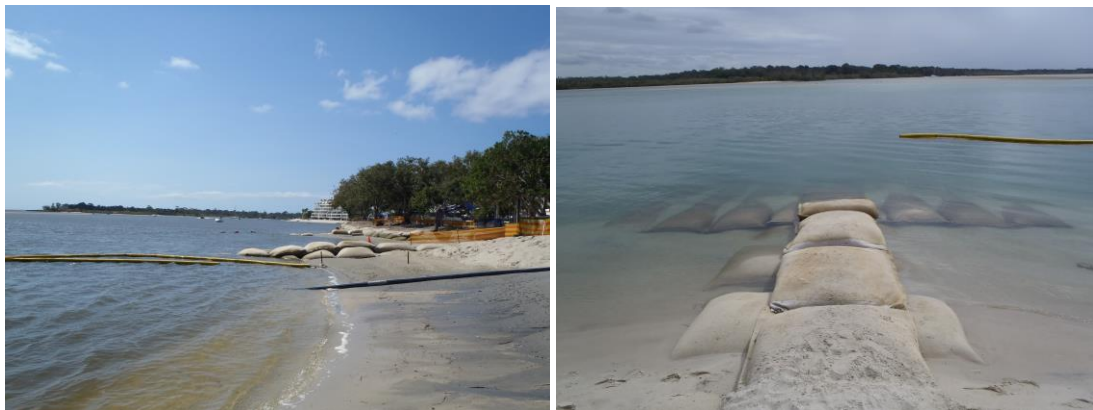
Figure 9. Completed Stage 1 Groyne
