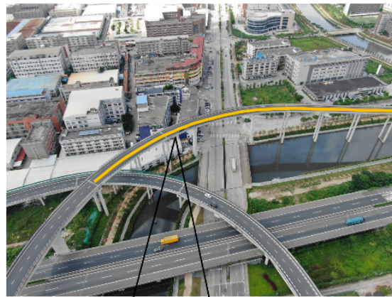
Ramp Bridge (Pier P27-P35)
