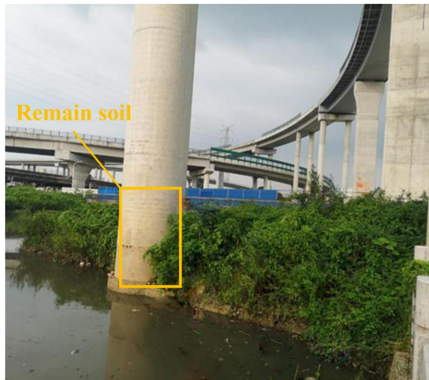
Figure 10. Surrounding conditions of Pier P30.
