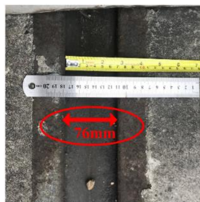
Expansion joint on Pier P33
