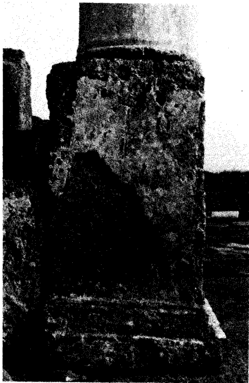
Figure 1. Deteriorated stucco of the Forum of Baelo Claudia.
