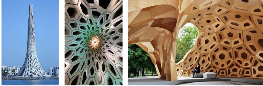
Figure 3: Hex-dominant structures. Left and Middle: The KAUST Breakwater Beacon at the entrance to the harbor of the King Abdullah University of Science and Technology in Saudi Arabia, by Urban Art Projects. Right: ICD/ITKE Research Pavilion 2011 at the University of Stuttgart.
