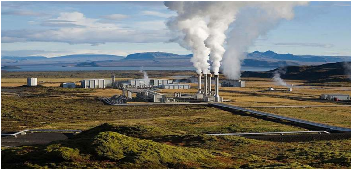
Fig. 3 Nesjavellir power station in Iceland, a central geothermal power plant [51, 52]
