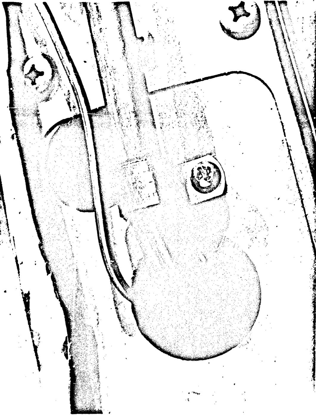
Figure 25. Antivibration Clamp, Oxidizer Line at Raceway Exit
