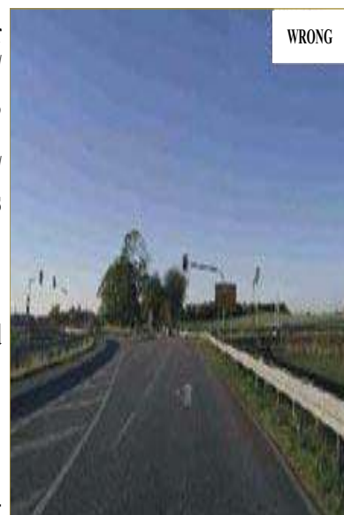
Figure 5: Junction, perceptible only at 100 m distance: the minor road seems to be the main road, unexpected braking and high speed at this point cause rear end and sideswipe collisions [16]
