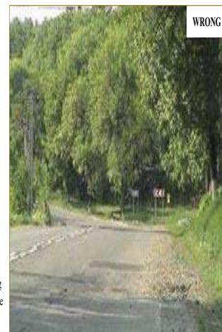
Figure 8: Course of the bend is not perceptible because inside bend is obscured: unexpected braking, steering manoeuvres and high speed cause drive off the road [23]
