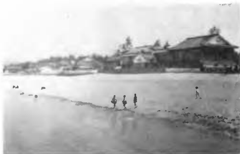
Fig.8 In 1957, the Kaike beach had been seen a stable wide sandy beach. The berm height of sandy beach in front of the seawall was nearly equal to that of the crest of the seawall.
