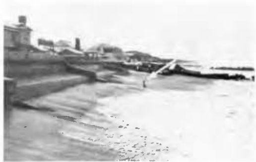
Fig.9 In December 1960, most of the sandy beach were vanished. The arrow mark on the center of the picture shows the fountainhead No.3 shown in Figure 4.
