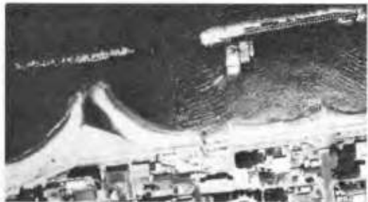
Fig.18 Aerial view of the Nos. 1 and 2 breakwater and tombolos by means of a radio controlled model plane.
