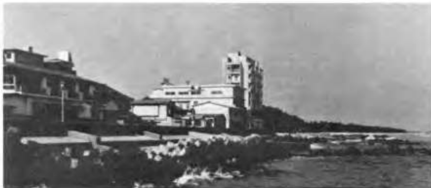
Fig.12 As the wave defence works, armour concrete blocks, named Hexa-leg block, were piled up in front of the seawall. But a number of these blocks have sank under the sea bed ( photo in 1970 ).
