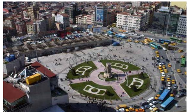
Fig. 24. Taksim Square before pedestrianizaing project [20].
