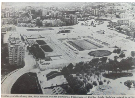
Fig. 10. Taksim barracks after its Demolition -Gezi Park [7].
