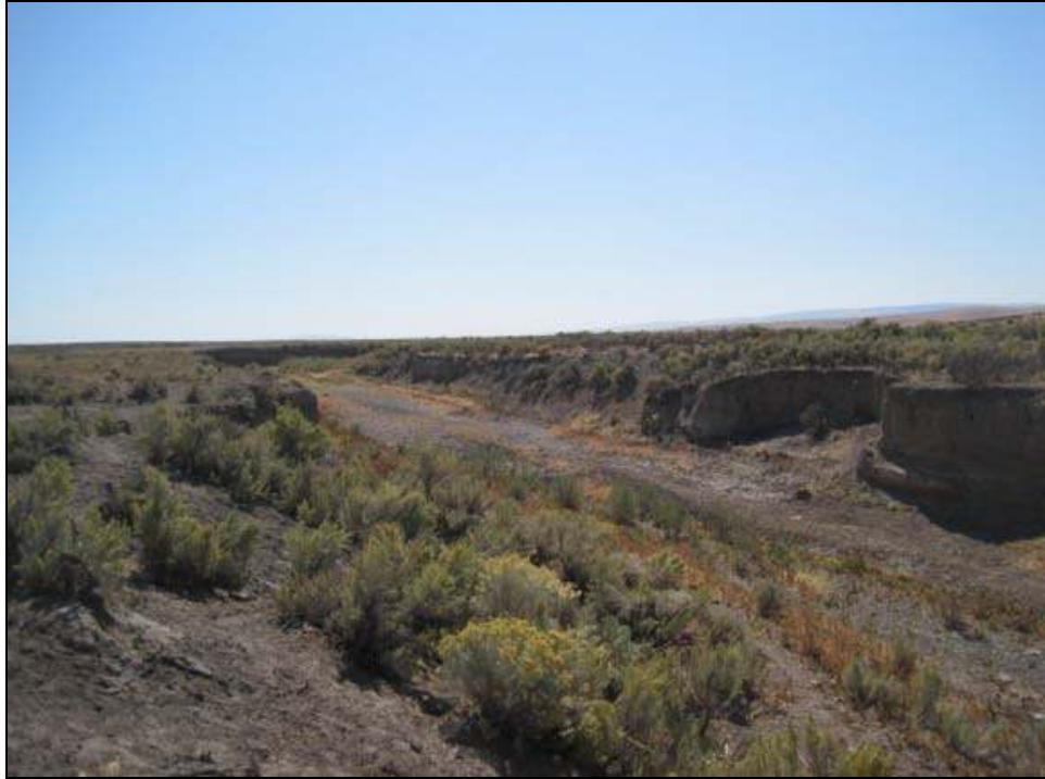
Figure 52. Active channel at McDermitt Creek, NV.
