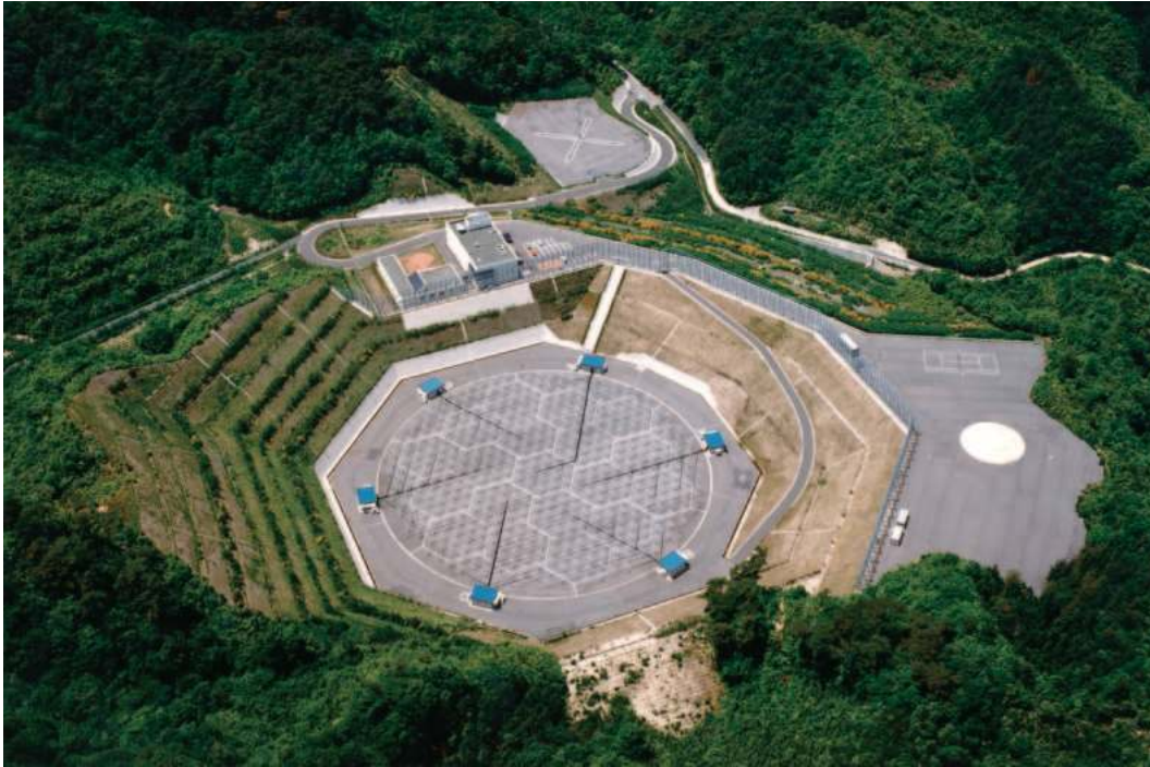
Fig. 1. An aerial photo of the MU radar operated by RISH, Kyoto University, in Shigaraki, Japan. The active phased array antenna has 475 Yagi elements and is 103 m in diameter.
