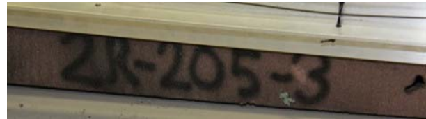
Fig. 12: Photograph of the panel identification number of the panel for documentation in the DCS.
