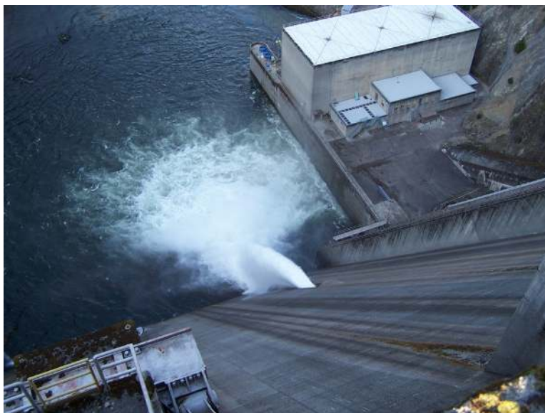
Figure 4.8. Regulating outlet discharge at Detroit Dam when the control gate was open 1 ft.
