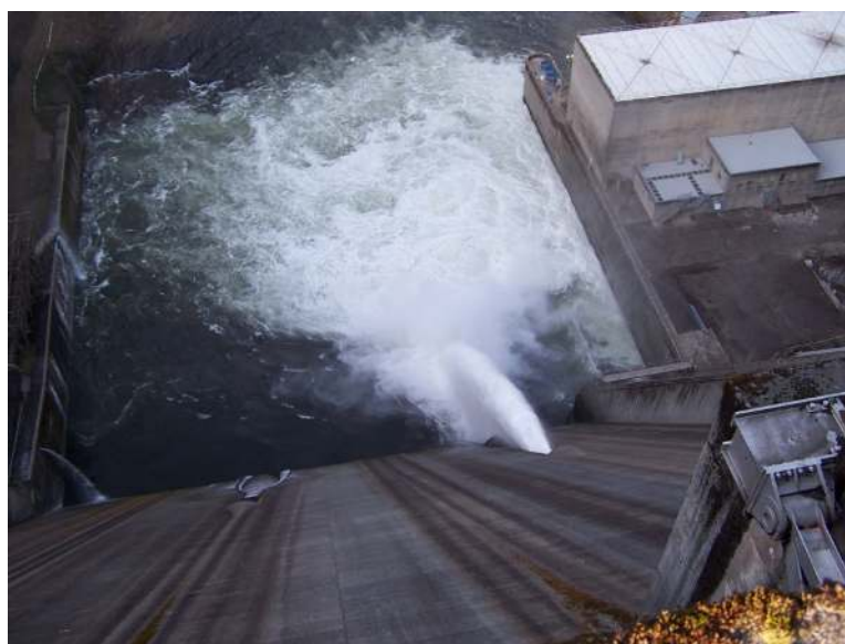
Figure 4.9. Regulating outlet discharge at Detroit Dam when the control gate was open 5 ft.
