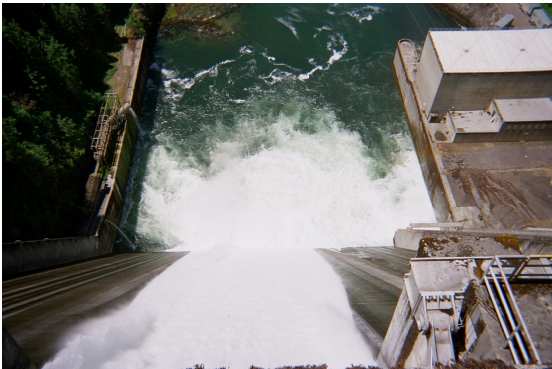
Figure 4.3. Flow through Spillbay 3, 1.5-ft gate opening (1560 cfs discharge) spreads to adjoining spillbays.
