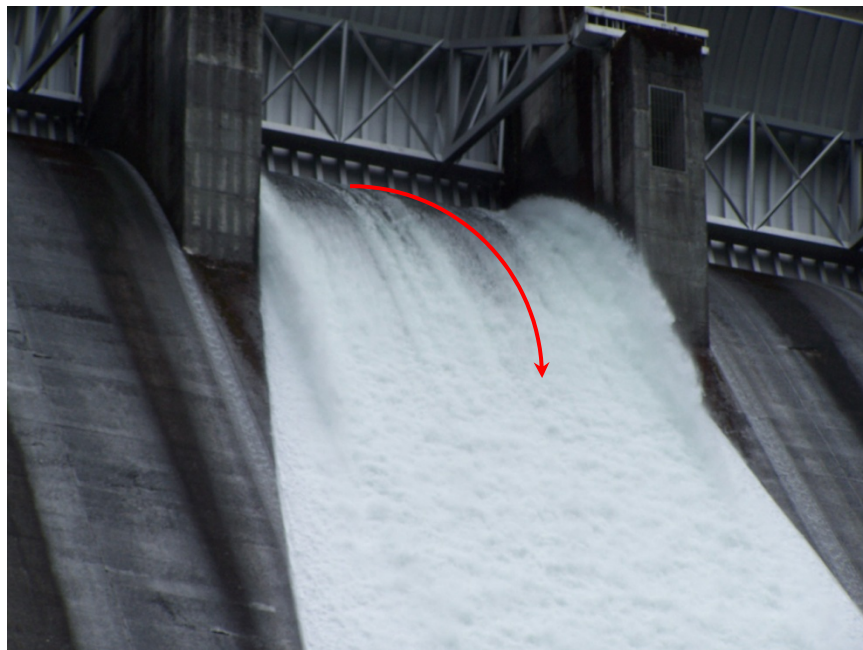
Figure 4.4. A hydraulic jump carries the Sensor Fish down the spillway chute as flow passes under the tainter gate in Spillbay 3 with the gate open 1.5 ft (1560 cfs discharge).
