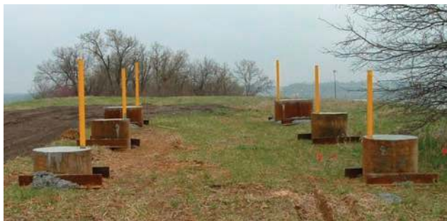
[FIG. 2a] Test Shafts
