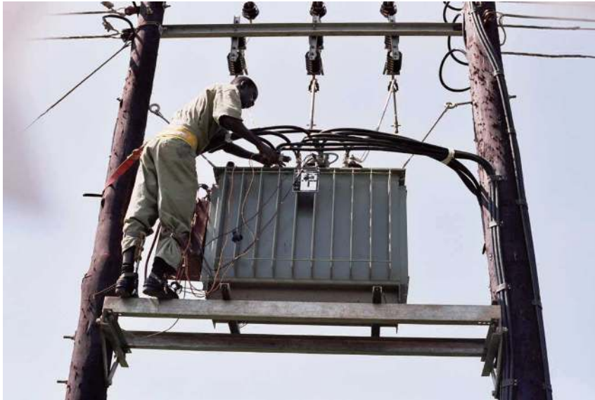
Figure 3.3: Technician installing instrument by the transformer
