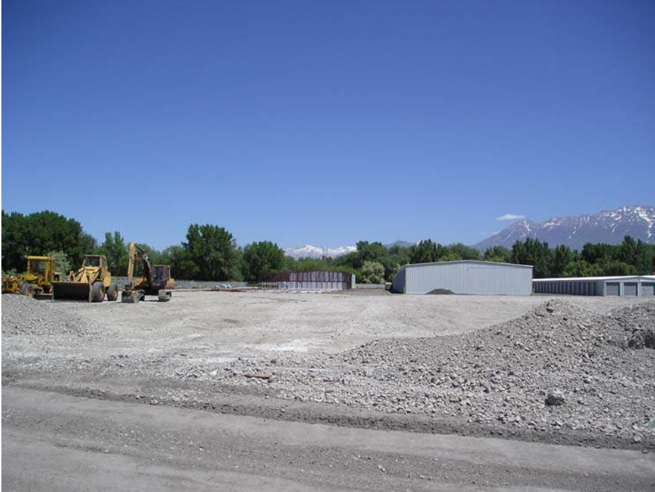
FIGURE 4-1 Unpaved recycled concrete material field site.
