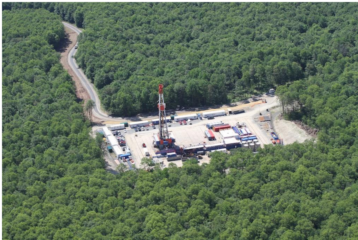
Figure 2.1 Aerial view of a typical hydraulic fracturing well site in the Marcellus shale basin, U.S. (Photo credit: Bill Howard—The Downstream Project, via LightHawk/SkyTruth).
