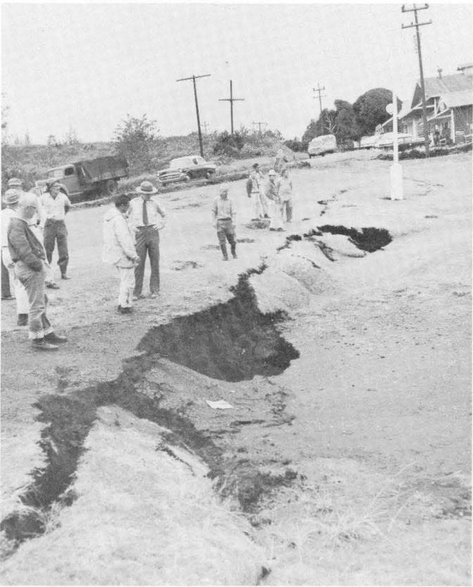
FIGURE 41.—Subsidence of the graben in the Kapoho area that occurred prior to eruption outbreak. Top : Koaie fault cuts the old railroad-bed road north of Kapoho. Picture was taken January 14 (day after faulting) and shows the fine-grained salty ash deposit spewed out by the steaming vents earlier in the morning. View is toward the northeast. Bottom : January 13, 1960. View westward along the Kapoho fault scarp in the village of Kapoho. Maximum vertical displacement is about 3\frac{1}{2} feet. Photographs by R. T. Haugen, National Park Service.
