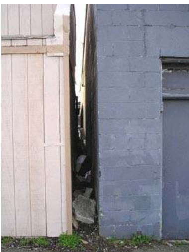
Figure 6.2 Another caretaking example. Courtesy of Seattle Neighborhood Group.
