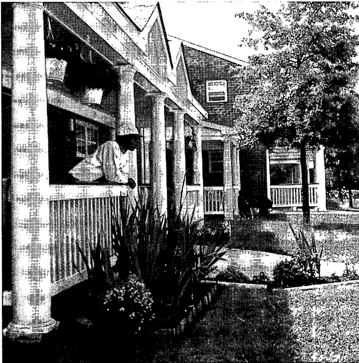
Diggs Town, Norfolk, Virginia, After the remodeling of the exterior that creates a neighborhood
