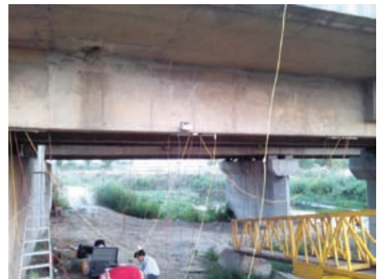
Figure 13: Photograph of the test site of Girder Bridge near Hapur.
