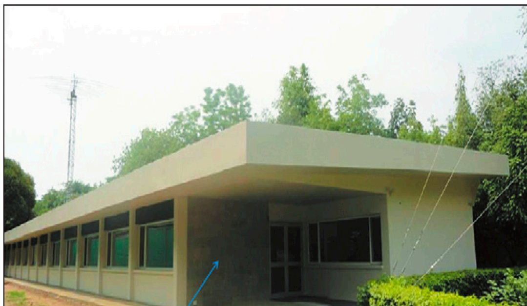
Figure 12. LC 3 AAC blocks used for an office building in the Swiss Embassy, New Delhi [76].
