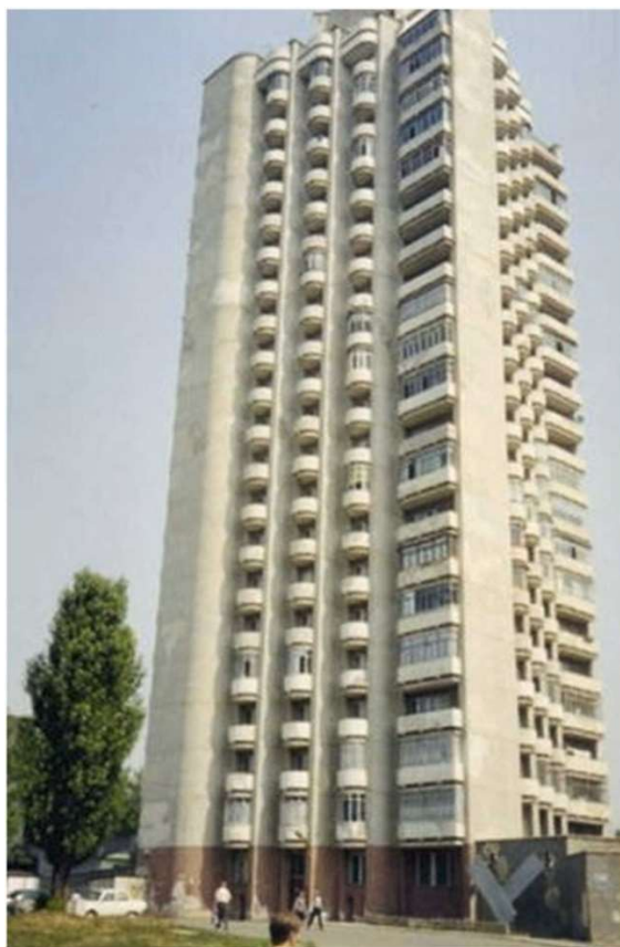
Figure 20. Residential building made using geopolymer concrete without any OPC in 1989 in Liepstk, the Russian Federation [93].
