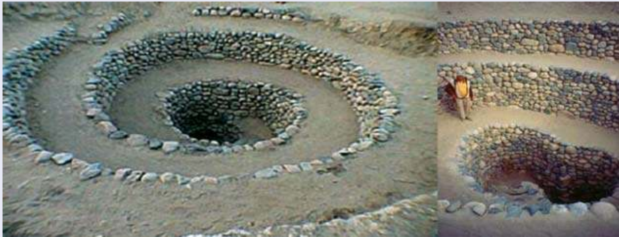
Figure 5.11: Nasca (southern coast of Peru) system of water cropping for underground aqueducts and feeding the phreatic layers.
