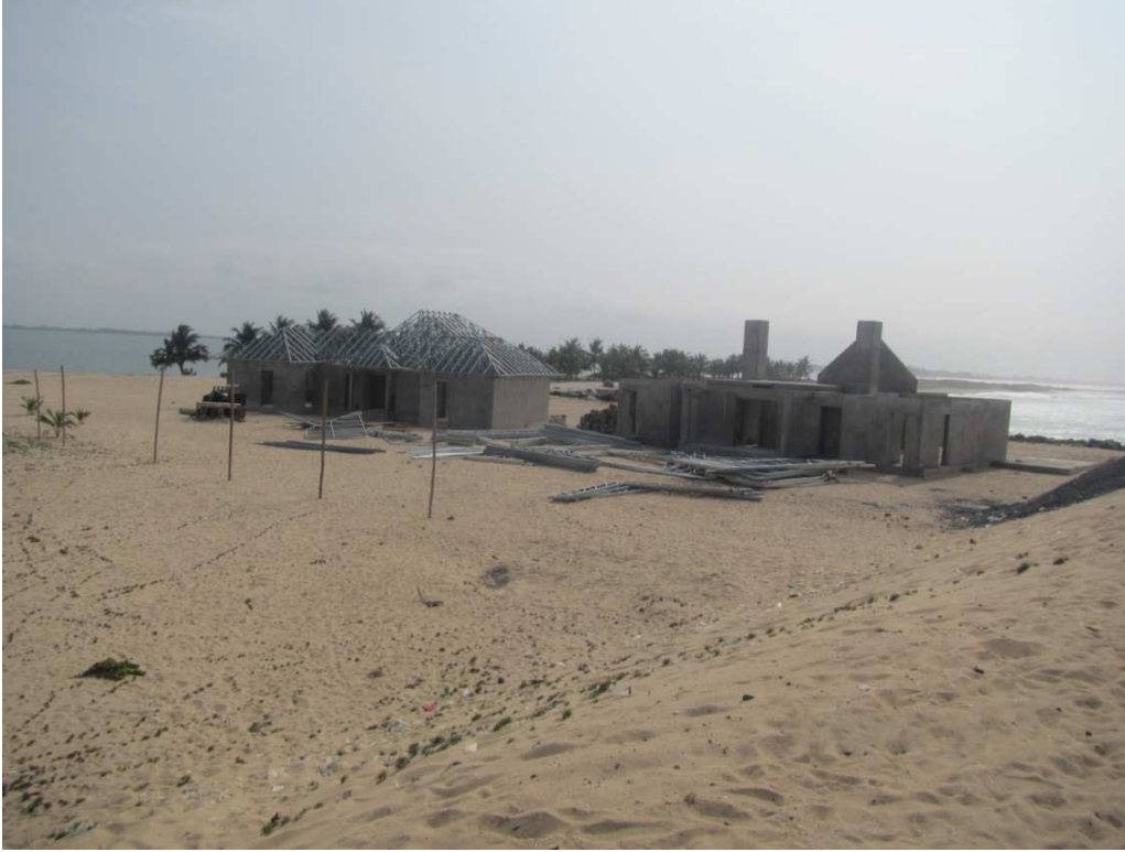
Figure 6.3 Trasacco Structures at the Volta River Estuary
