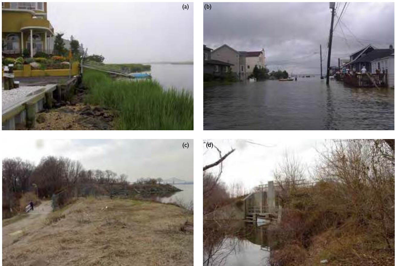
Figure 11.4 Vulnerability of New Jersey's coastal zone. (a) Wetland fringe lacks room for wetland migration (Monmouth, August 2003). (b) Low bay sides of barrier islands are vulnerable to even a modest storm surge (Ship Bottom, September 2, 2006). (c) Gibbstown Levee and (d) associated tide gate protect lowlying areas of Greenwich Township (March 2003) [Photo source: ©James G. Titus, used with permission].
