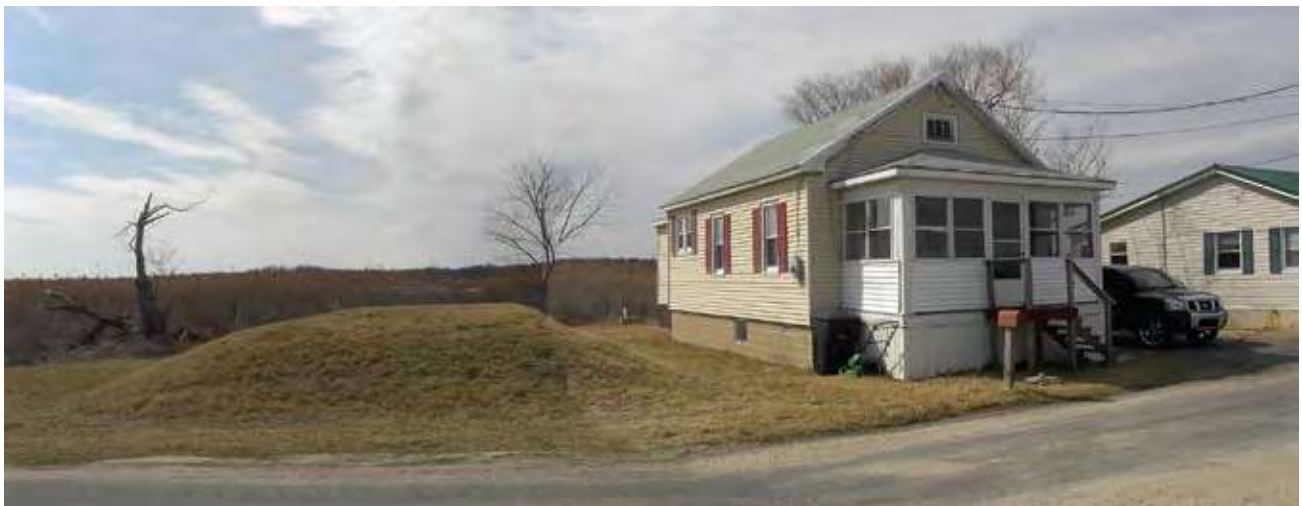
Figure 12.9 Mounds-based septic system next to house along the back side of Pickering Beach, Delaware (March 2009). [Photo source: ©James G. Titus, used with permission].
