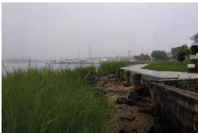
Figure 10.4 Wetland migration thwarted by development and shore protection. Elevating the land surface with fill prevents wetlands from migrating into the back yard with a small or modest rise in sea level. The bulkhead prevents waves from eroding the land, which would otherwise provide sand and other soil materials to help enable the wetlands to accrete with rising sea level (Monmouth, New Jersey, August 2003) [Photo source: ©James G. Titus, used with permission].
