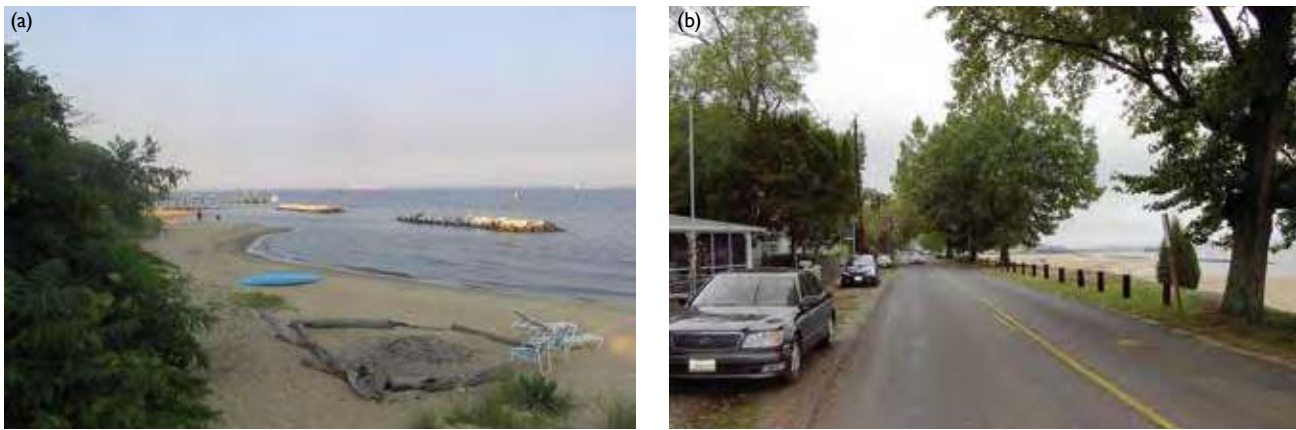
Figure 12.2 Beach nourishment along estuaries. (a) The Department of Natural Resources provided an interest-free loan to private landowners for a combined breakwater and beach nourishment project to preserve the recreational beach and protect homes in Bay Ridge, Maryland (July 2008). (b) The Virginia Beach Board and Town of Colonial Beach nourished the public beach along the Potomac River for recreation and to protect the road and homes to the left (October 2002) [Photo source: ©James G. Titus, used with permission].
