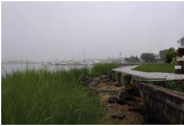
Figure 5.2 Fringing marsh and bulkhead, Monmouth County, New Jersey (August 2003) [Photo source: ©James G. Titus, used with permission].
