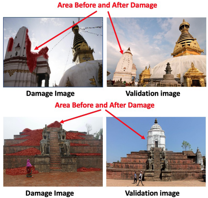
Fig. 9. Examples of ground truth damage area annotation.
