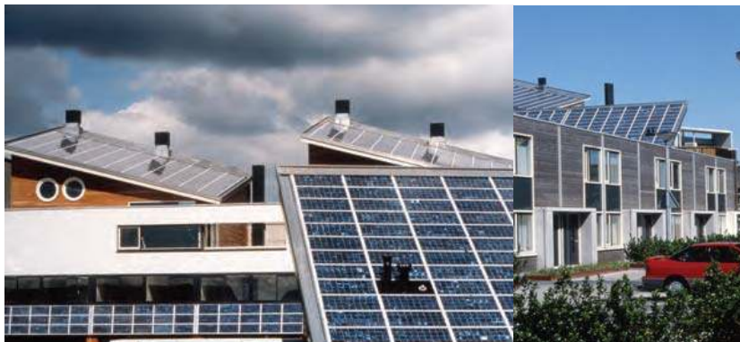
Figure 9 Examples of projects of Nieuw Sloten, Amsterdam.
