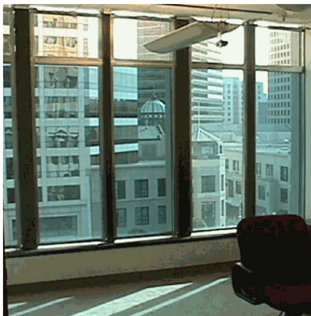
Fig. 7. Electrochromic windows installed in a test room (adapted from [50]).
