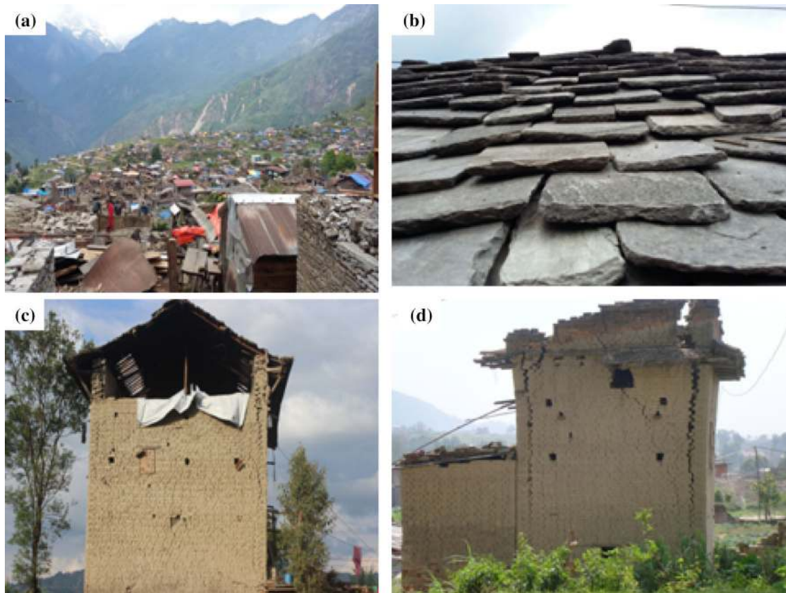
Fig. 16 a Heavily damaged neighborhood of Barpak village where 1250 houses out of 1450 total were collapsed. b Heavy stone roofing in Barpak. c Gable collapse in adobe house in Bhaktapur. d Separation of diagonal walls in an adobe house
