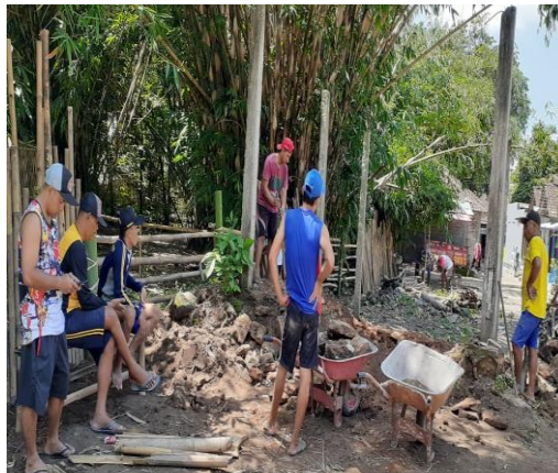
Figure 3. The Construction Process of the Taman Teak Larangan Open Stage
