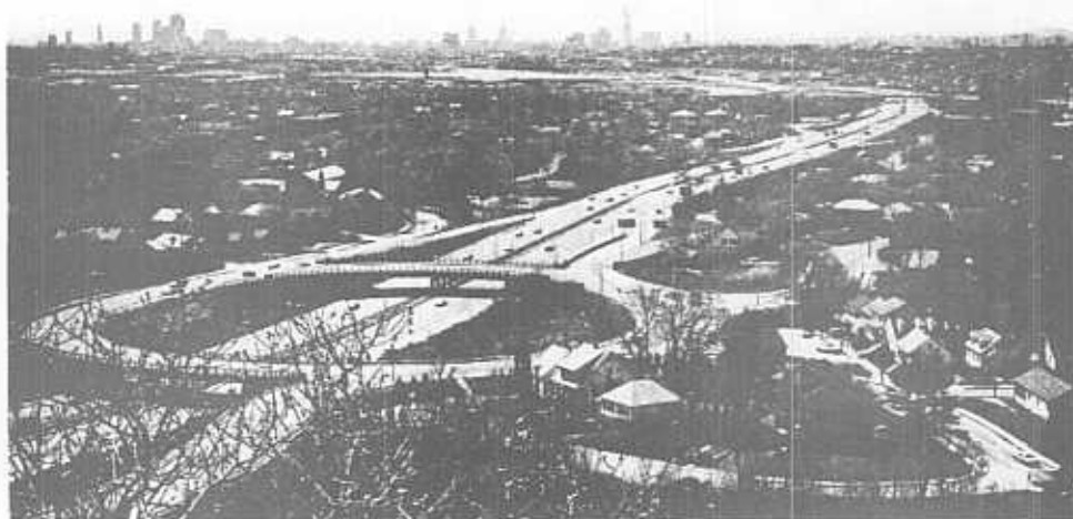
Figure D-10. Interstate Route 93 in Medford Facing South from a Lookout Tower Near Grid 6-7
