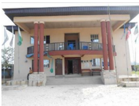
Plate 1. Showing Town Hall Project embarked upon by Community Development Committee (CDC) in Otari community in the study area Source: Authors' field survey, 2016
