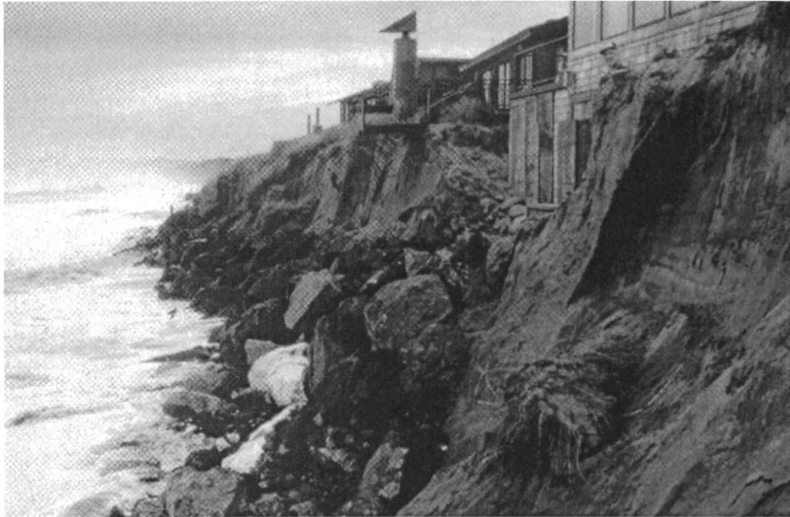
Figure 3. Beach and dune erosion at the Pajaro Dunes development in early 1983. Over 15 m of the dunes were eroded during the storms of early 1983, undermining the foundations of many structures. The rip-rap was emplaced at the height of the storms to stop further erosion and the possible collapse of structures.
