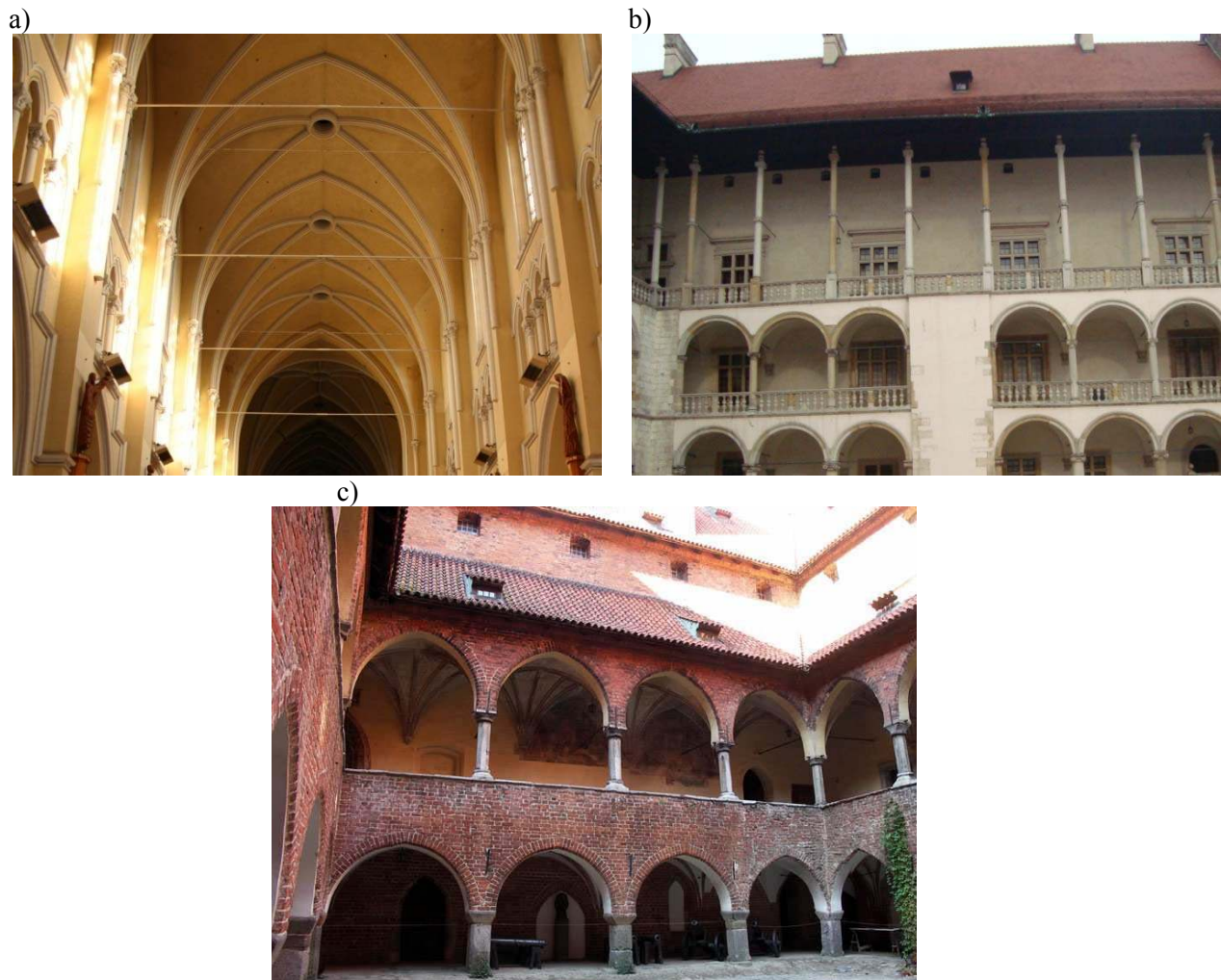
Fig.1. Examples of tie-rod usage in brick arched structures: a) The Cathedral Basilica of the Holy Family in Częstochowa, b) the cloisters of the Wawel Royal Castle, c) the cloisters of the Castle in Lidzbark Warmiński.
