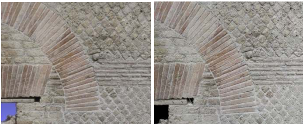
Figure 4. Visual comparison between the Photogrammetric mesh model (left) and the coloured scanner point cloud (right). It is interesting to point out that the density of the point model is so high that the difference between the laser and the photogrammetric model is almost irrelevant, allowing to clearly distinguish every details of the façade on both models
