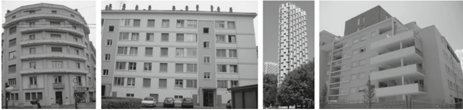
Fig. 2 Examples of considered RC shear walls buildings in Grenoble constructed from left to right in the 1930s, 1950s, 1960s and the years 2000
