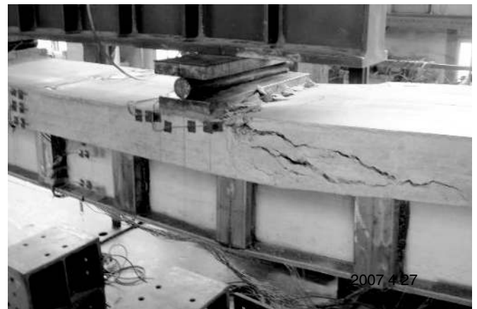
(a) Compression failure of concrete deck
