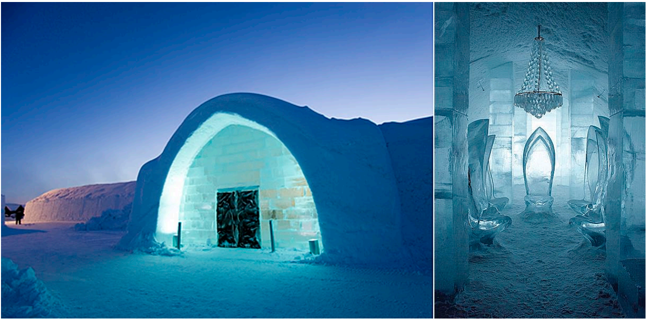
Figure 2. The exterior (left) and interior (right) of the Icehotel. The basic building material is frozen water.
