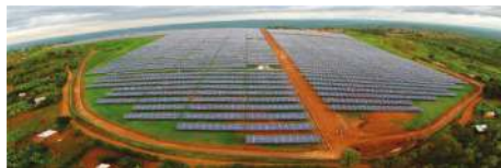
FIGURE 12: The Rwamagana solar power station [53].
