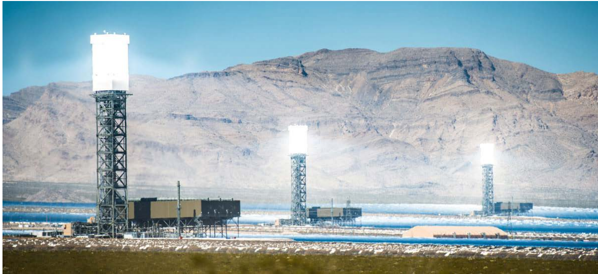
Figure 6-2. Ivanpah water/steam receivers Source: Google Images
