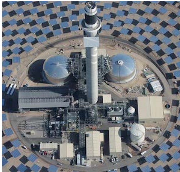
Figure 6-5. Two-tank thermal storage system at Crescent Dunes Source: Google Images
