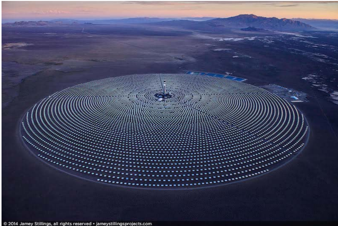
Figure 6-4. Crescent Dunes heliostat-field layout for salt receiver Source: Google Images
