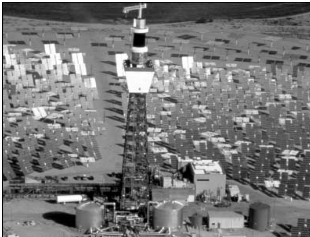
This concentrating solar power tower system — known as Solar Two — near Barstow, California, is the world's largest central receiver plant.
