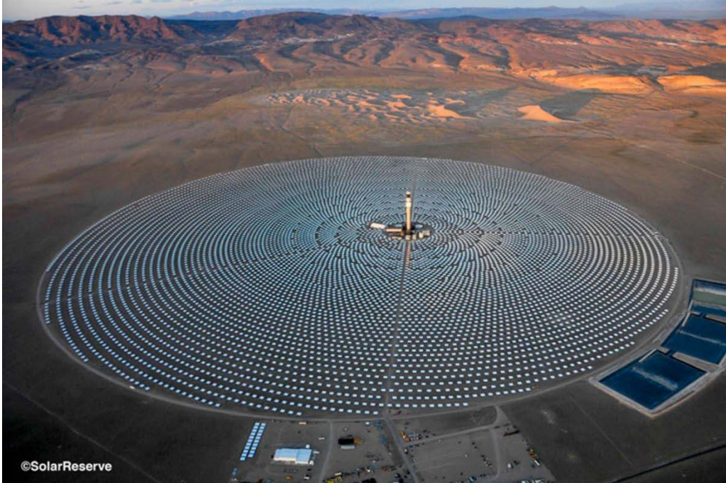
Figure 5. 110-MW e Crescent Dunes Solar Energy Project in Tonopah, Nevada, with 10 hours of thermal storage. (source: SolarReserve)
