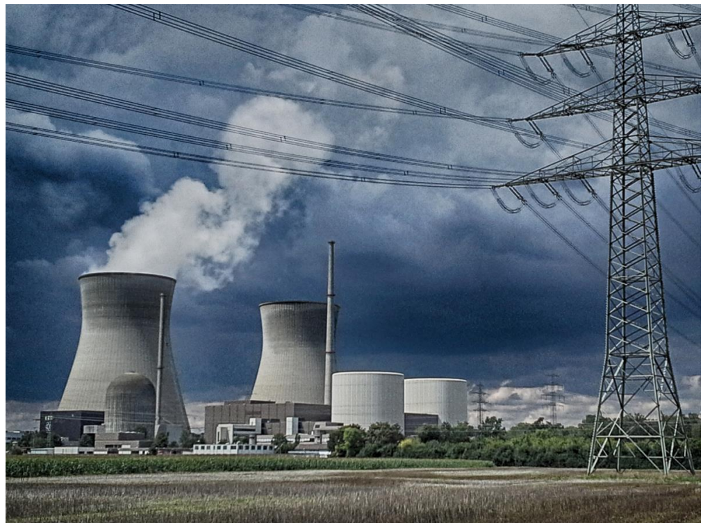
Figure 1. Nuclear Powerplant Gundremmingen, Germany (Photo Dirk HR Spennemann, August 2014).
