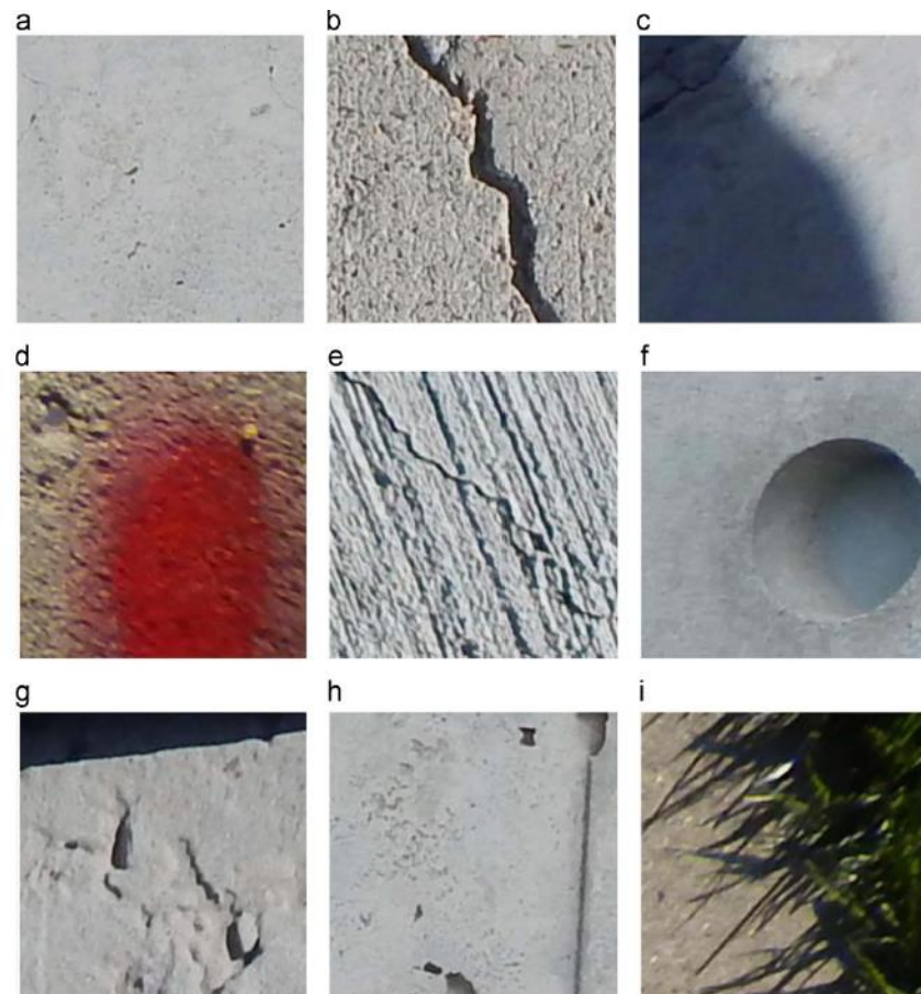
Figure 12. SDNET2018 images include (a) fine cracks, (b) coarse cracks, (c) shadows, (d) stains, (e) rough surface finishes, (f) inclusion sand voids, (g) edges, (h) joint sand surface scaling, and (i) background obstructions.
