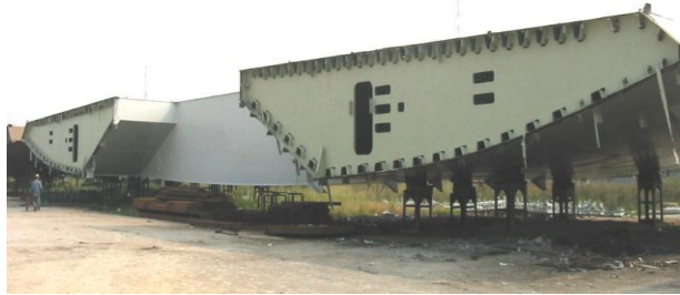
Figure 3: Typical steel deck segment of the bridge
