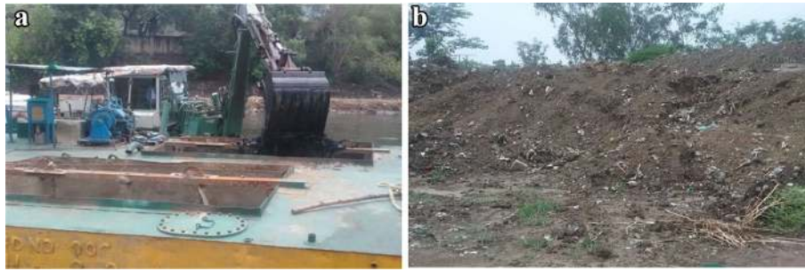
Fig. 1 a Dredging of Nazafgarh Drain. b Dumping of dredged soils along banks
