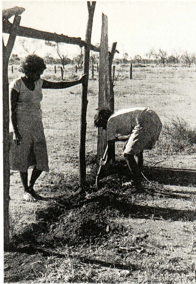
Plate 8.5: Hilda and June Bird construct a new alwekere at Angkwele outstation.
